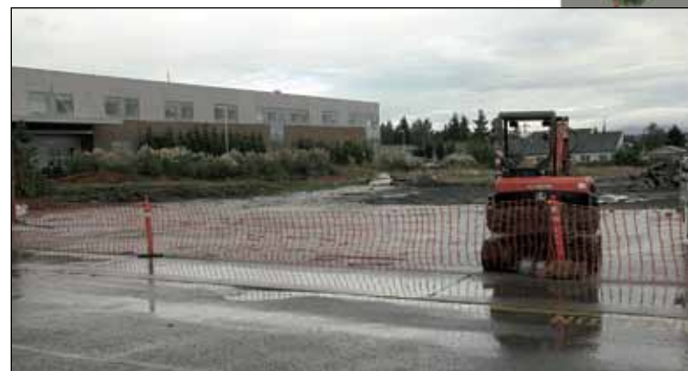
Site preparation begins for the Medical Arts Pavilion.
