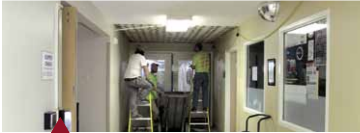
Workers remove old ceiling materials outside the main hospital storeroom.
