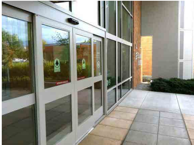
Multiple entries and wayfinding systems do not support an easy navigation
