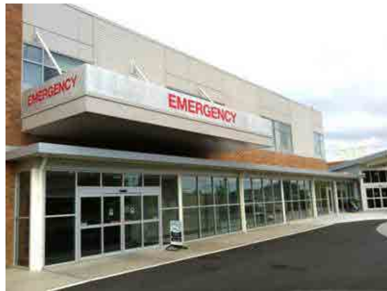
Designed discharge area underutilized despite proximity to parking/pickup space, patient preference is to use either the Main or ED entry – requires additional steps and communication in the discharge process
